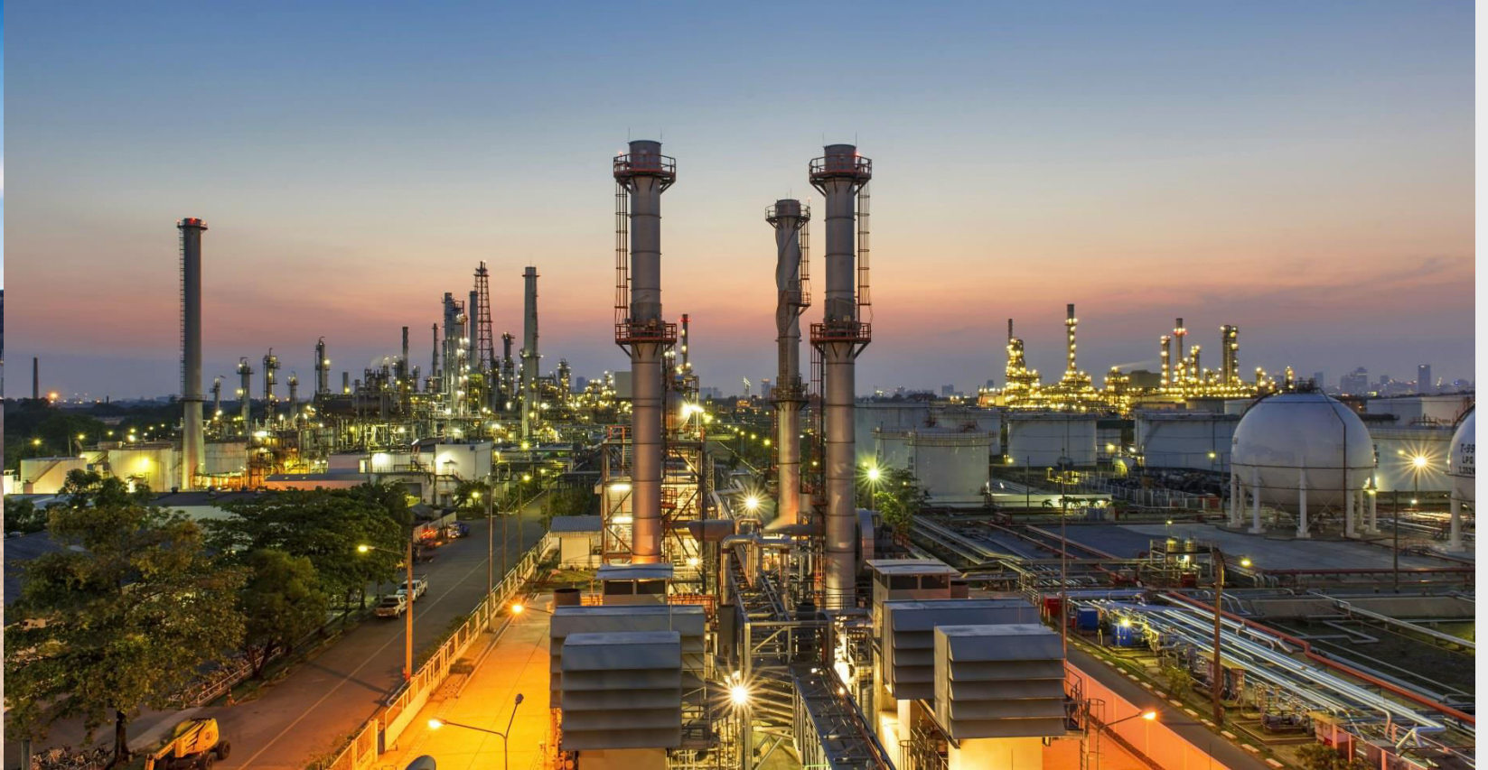
Data center fuel?
